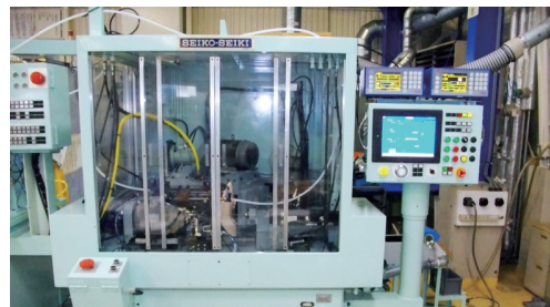
After overhaul and retrofit
