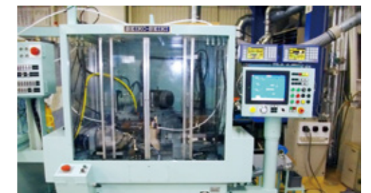
After overhaul and retrofit
